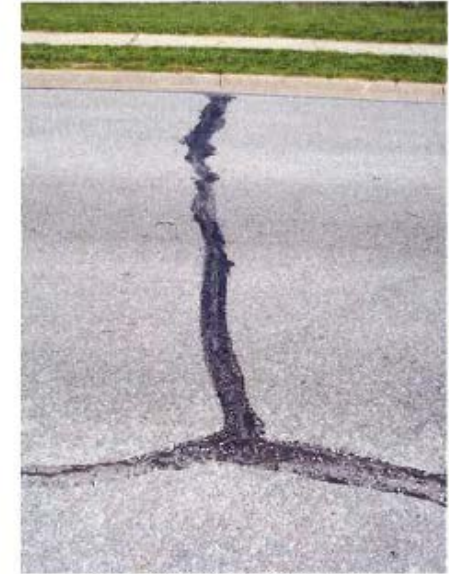
Effectively Sealed Cracking
