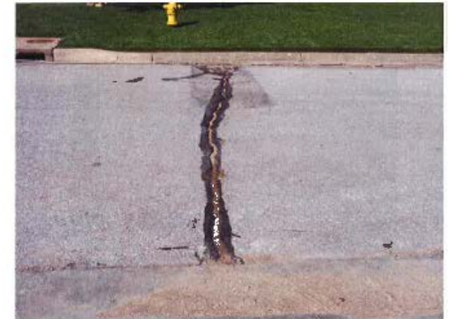
Cracking Not Effectively Sealed
